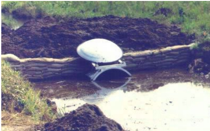
Figure 1. 36" Flap gate on Coastal North Carolina drainage canal. Photo by Doug Newcomb/FWS
