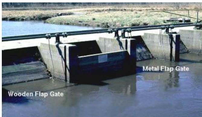
Figure 2. Water control structure with metal and wooden flap gates.
